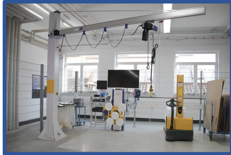
Jib Crane & Hoist
